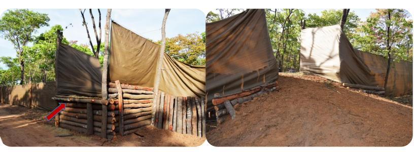
To eliminate the potential gap (see red arrow above) between the truck opening and the offloading ramp, an extra pole or piece of conveyor belt may be used.
