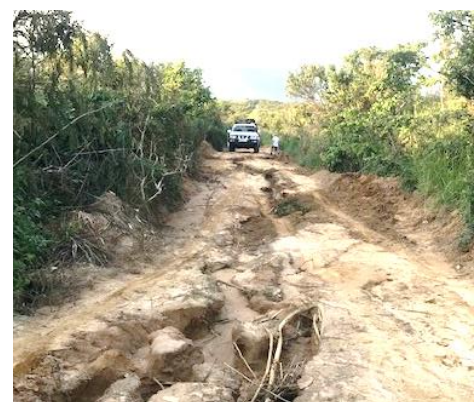
Figure 19 Heavily eroded road in the DRC due to flash floods and bad maintenance (photo © U. Tubbesing)
